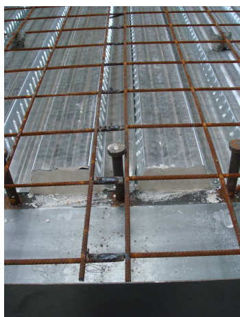
a- Welded reinforcement joint prior to the concrete casting
