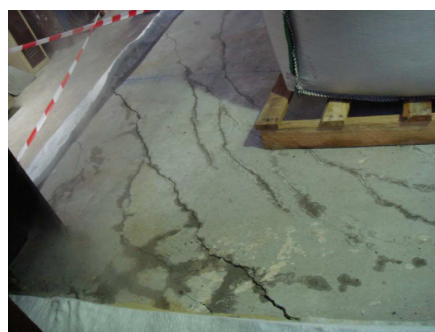
b- at the end of fire test
