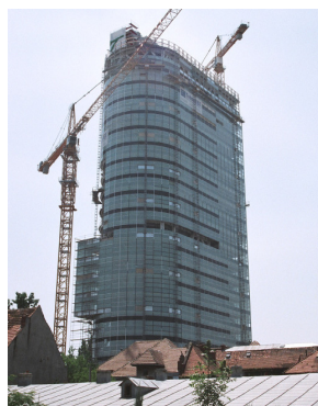
Fig. 7 - Photo during construction
