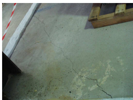
a- at the beginning of fire test
