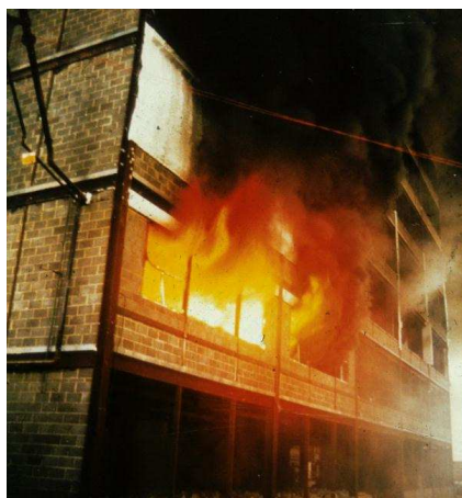
Fig. 2 – One of the fire tests on Cardington building
