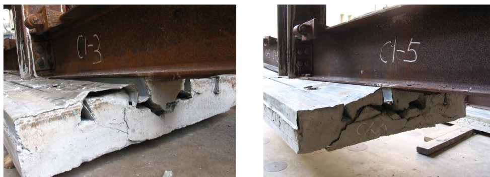
Figure 13. Local detachment of shear stud of C1-3 & C1-5 specimen
