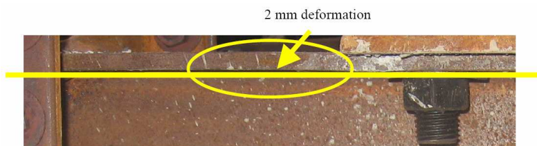
Figure 11. Buckling of beam bottom flange for C1-1
