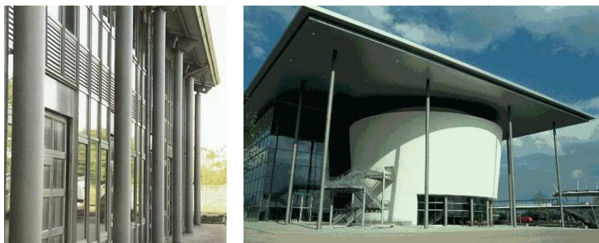
Fig. 1 - External application of slender concrete-filled steel columns © Stahl + Verbundbau .
