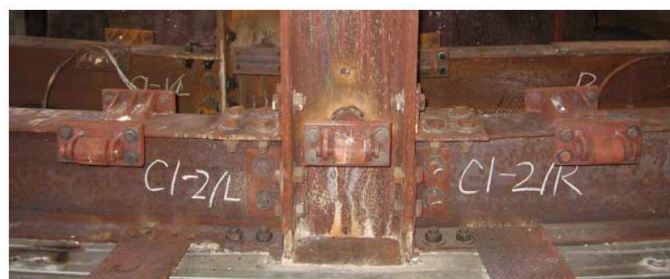
Figure 8. Local view of C1-2
