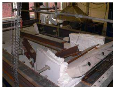
(b) Collapse of Slab T3
