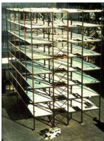
Fig. 1 – Cardington test building prior to concrete casting of the floor
