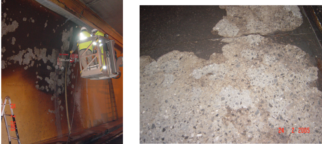
Figure 1. Local explosions in the concrete walls of the tunnel after fire.
