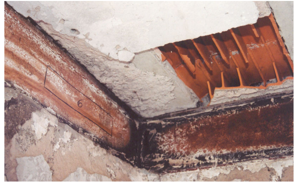
Fig. 4 – Apartment's plant with furniture, Fig. 5 – Composite slab damage detail. showing where the fire started.
