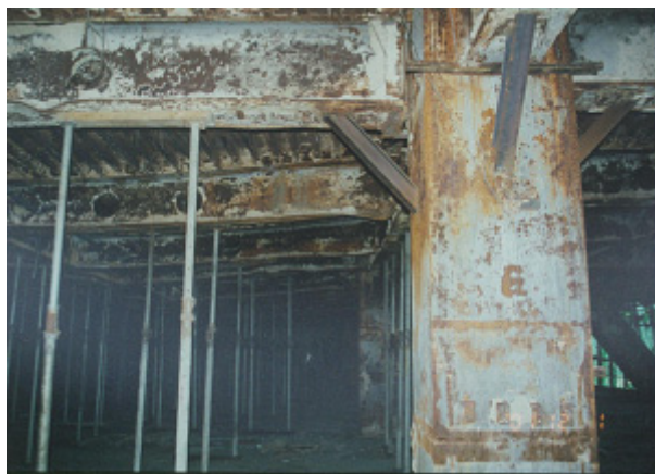
Fig. 1 Damages to beam-column connections in Taipei Science and Technology Park
