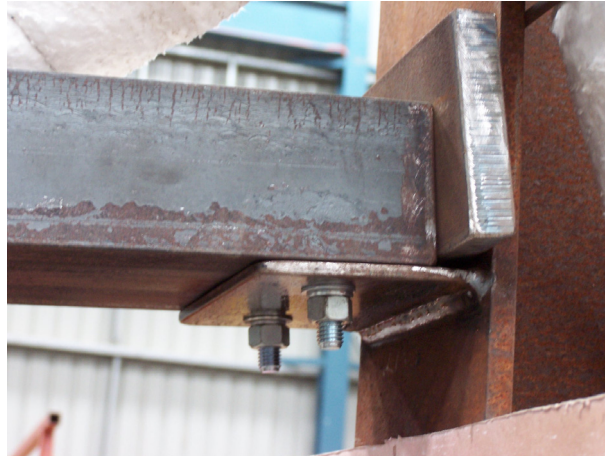
Figure 3 : Photograph of End Connection
