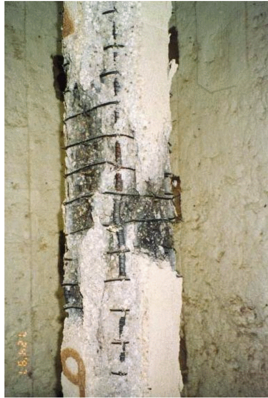
Modified Tie Configuration
