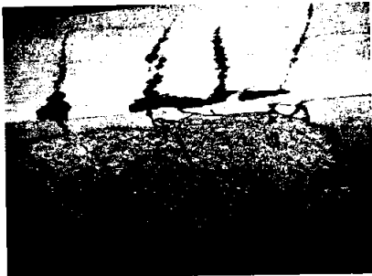
Figure 4. Cracks on an unloaded small slab.
